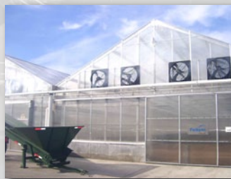
Solar Sludge Drying Area
